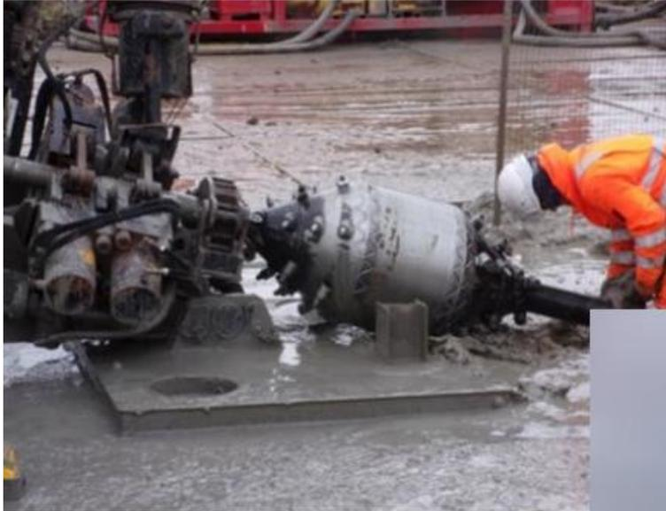
End of directional drill reaming bit appearing from the bore
