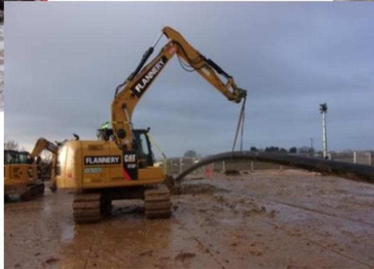
The 320 metre sewer pipe being pulled through the directional drill sleeve
